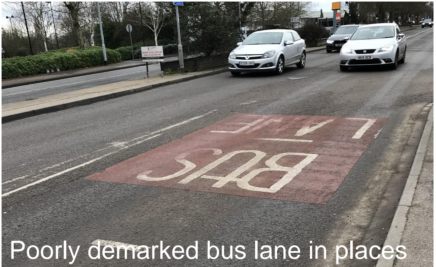
Figure 4.5: Bus Infrastructure on Newmarket Road
