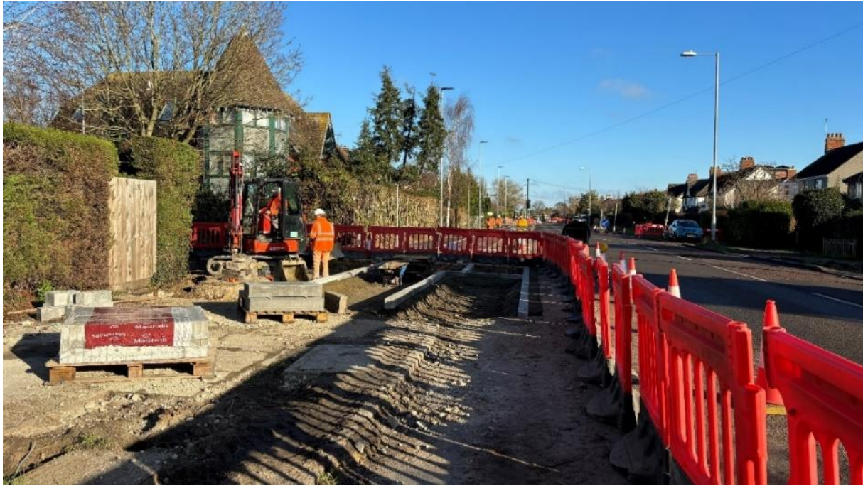
Photo: Construction at Downham's Lane
