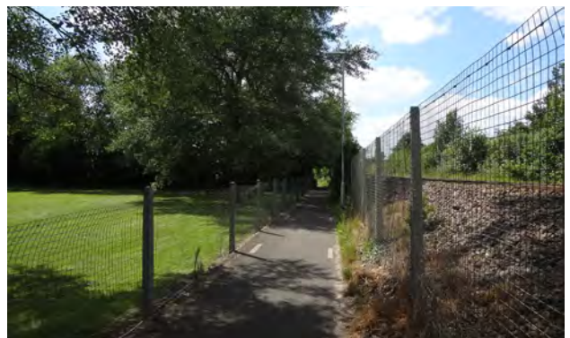
Existing shared cycle path from Fulbourn Old Drift to Yarrow Road along the railway
