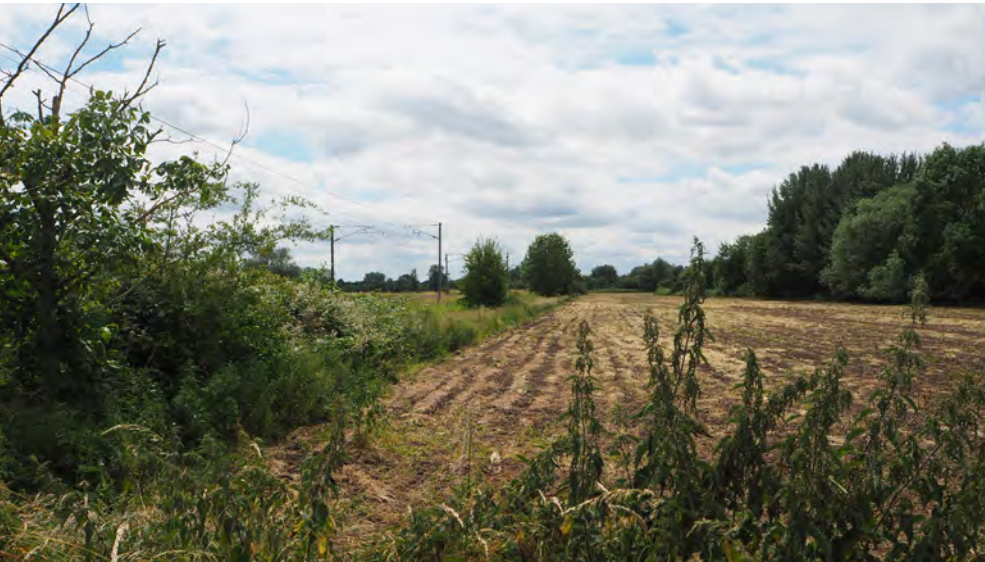
Existing stretch of railway, ditch and fields from Cambridge North to Waterbeach Station
